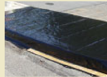
4. (above) Concrete is leveled with a screed.
