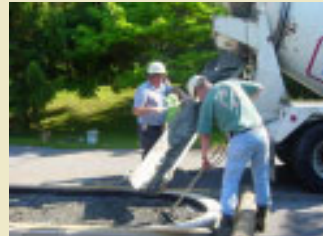
3. (above) Concrete is poured and spread.
